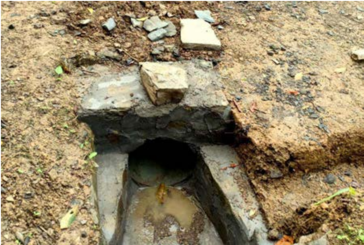
20. Repair of irrigation channel for WTRC.
