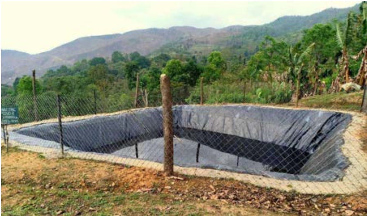
5. Fence Reconstruction cum Water Harvesting Structure.
