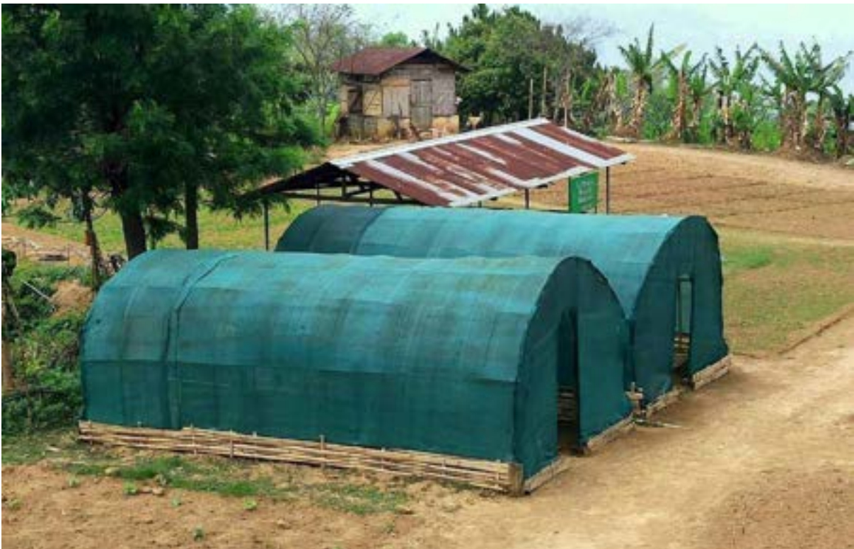
19. Renovation of Nursery Green House.
